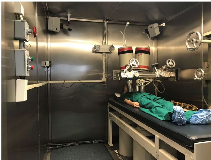
Figure 9.1. The Whole-Body counting facility at CEMRC
