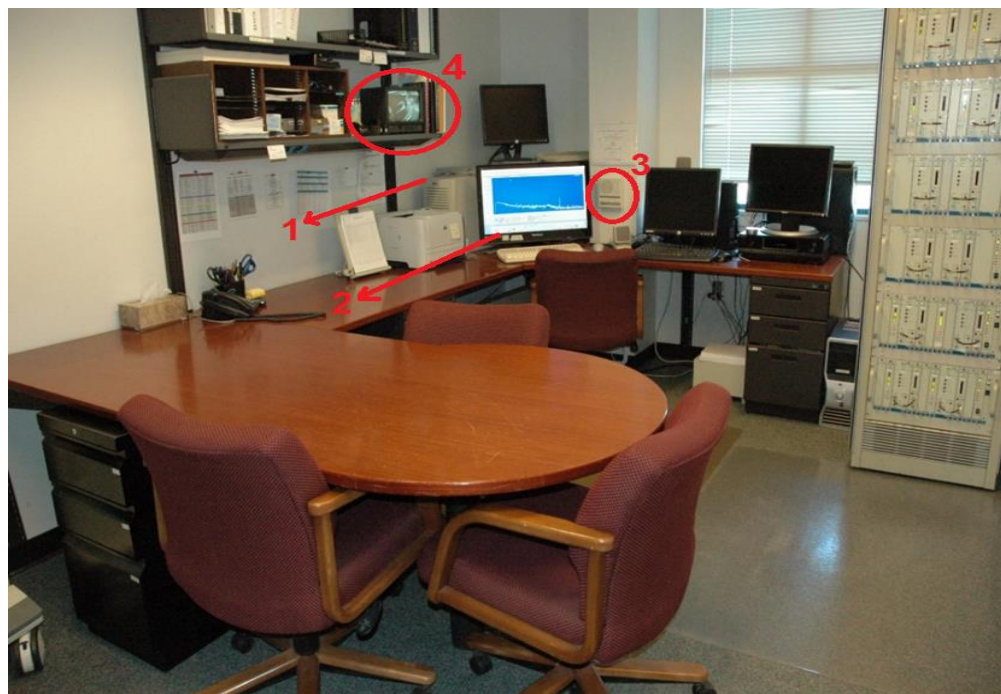
Figure 7.4. Operator's control room: (1) instrument control workstation, (2) computer monitor display, (3) intercom (4) video display terminal.
